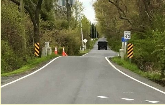
Prior to the Work
