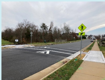
Raised Crosswalk at Lennox Hale Drive
